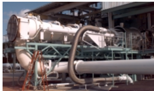
Figure 11: Pratt & Whitney E-8 Vacuum Test Facility
