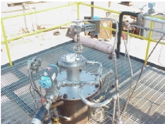
Figure 6: RL60 Ignition Rig Testing
